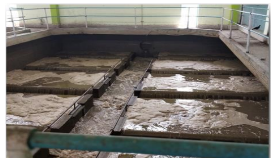
Figure 2 Rapid Sand Filter
